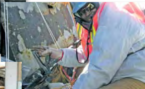
A Power Cable Maintainer splices control cables just days before the May 30th re-opening of the line.
