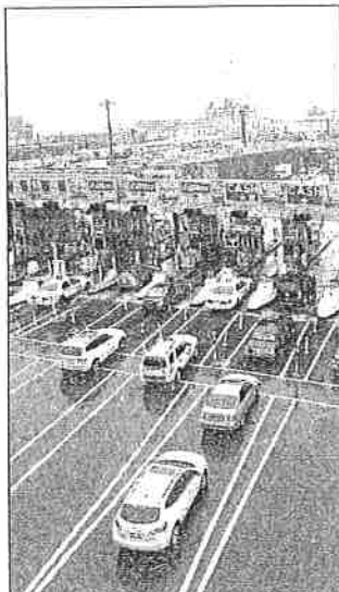
Aerial view of Manhattan-bound entrance of Queens-Midtown Tunnel, which is not manned by security on weekends. Photo by Andrew Theodorakis/Daily News
