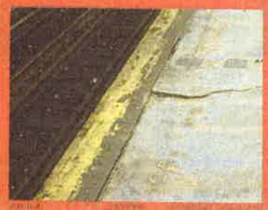
Above: Missing tile at the Fordham Road stop of the B/D trains. Below: Floor cracks at the Pelham Parkway stop on the 5 train.
