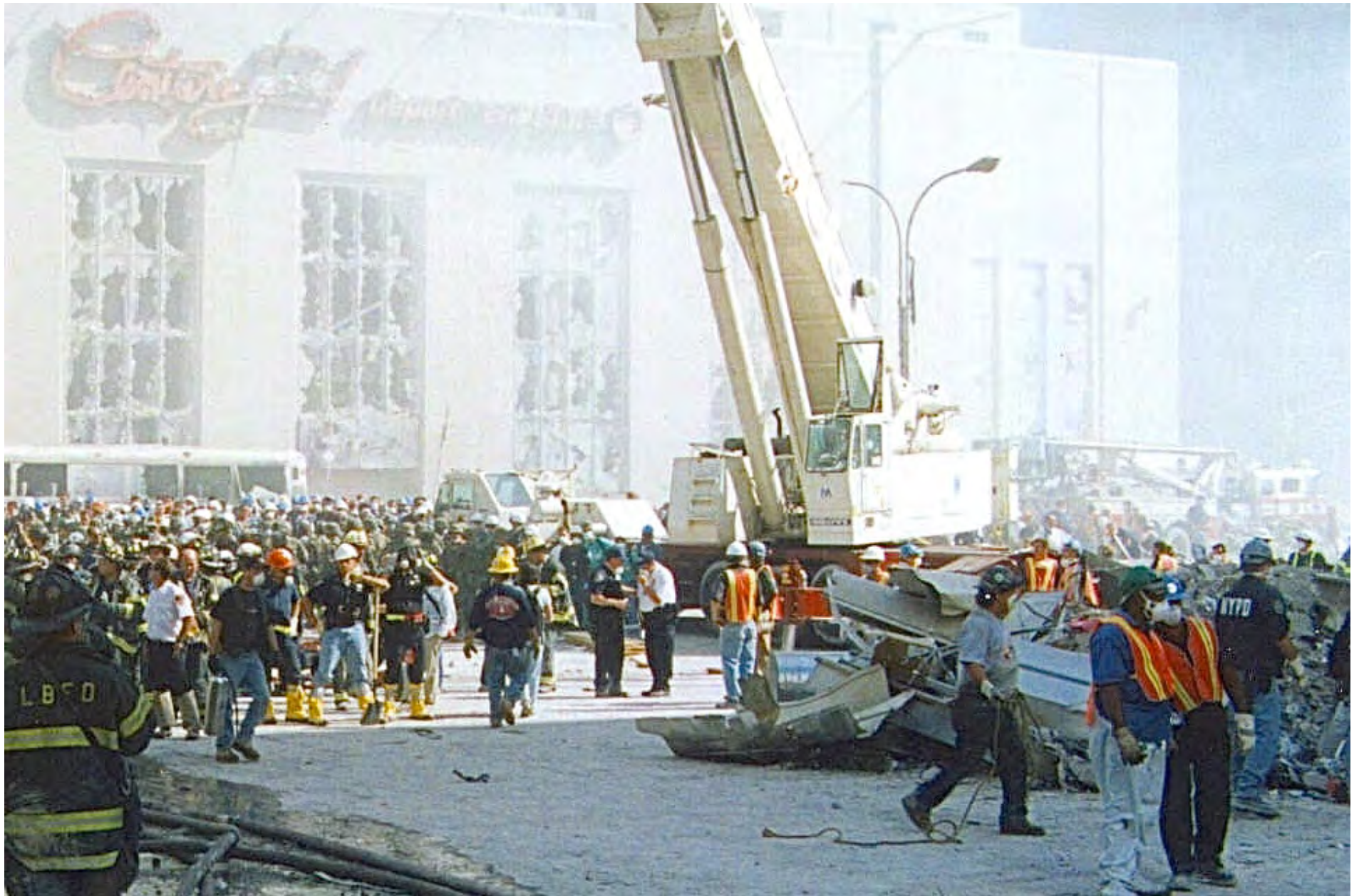
Crowd of rescuers. In the center, the biggest piece of equipment at Ground Zero was Transit's 100-ton Terex crane, normally used for lifting subway cars off of elevated structures.
