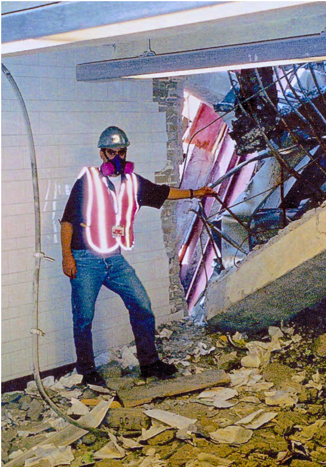
Electronic Equipment Maintainer Mario Galvet inspected the damage done to communications cables at the site. The cable at left, which was severed by the collapsing towers, originally extended through the WTC concourse. Mr. Galvet and other TA communications personnel, in cooperation with cellphone carriers, used this antenna during the rescue and recovery effort to attempt to activate the cellphones of victims lying underneath the rubble of the towers.
