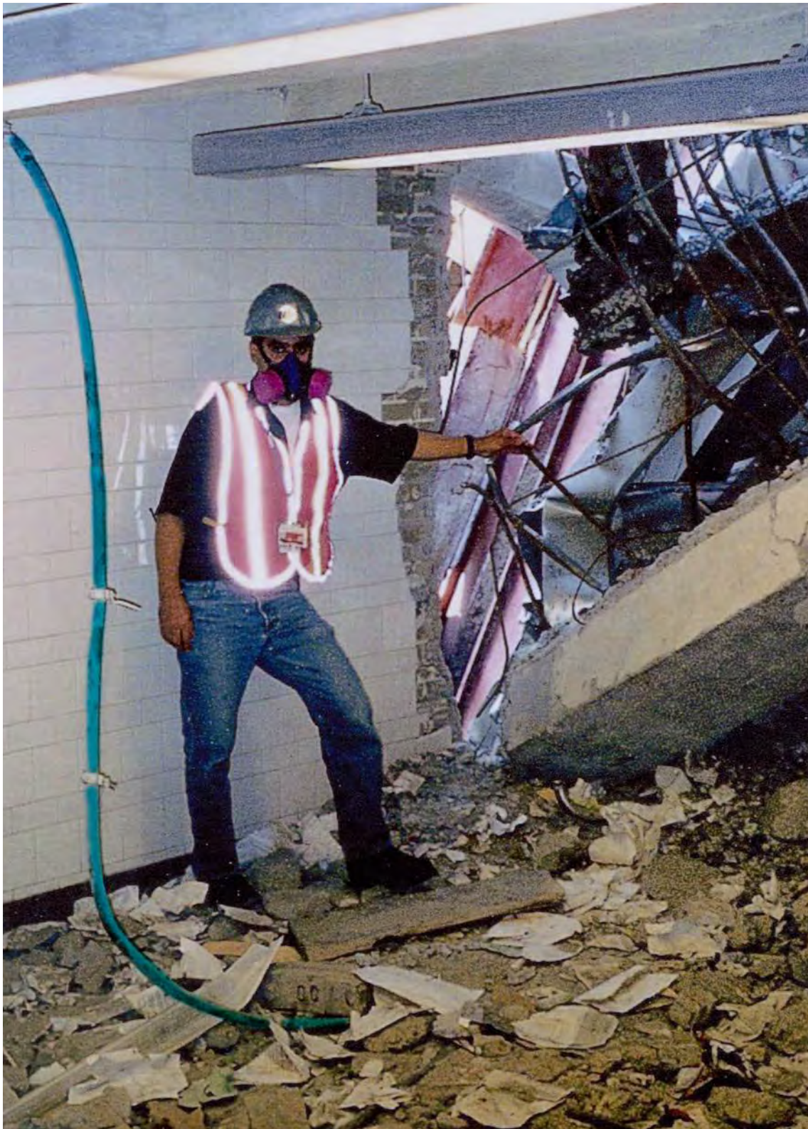
Electronic Equipment Maintainer Mario Galvet inspected the damage done to communications cables at the site. The cable at left (highlighted in blue), which was severed by the collapsing towers, originally extended through the WTC concourse. Mr. Galvet and other TA communications personnel, in cooperation with cellphone carriers, used this antenna during the rescue and recovery effort to attempt to activate the cellphones of victims lying underneath the rubble of the towers.
