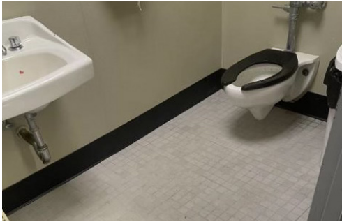
Renovated bathroom at Brighton Beach
