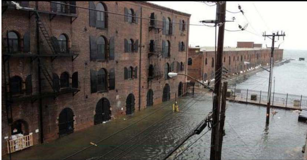
Hurricane Sandy Flooding, Red Hook 10.29.12 Photo: FDNY Incidents
