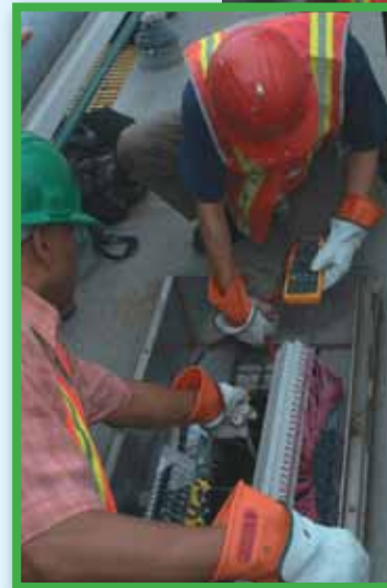
As Coney Island's Wonder Wheel rotates in the background, Local 100 members (above) take part in photovoltaic training, and (left) Simon Oui takes a meter reading to see how much current the panels are generating on a cloudy day.
