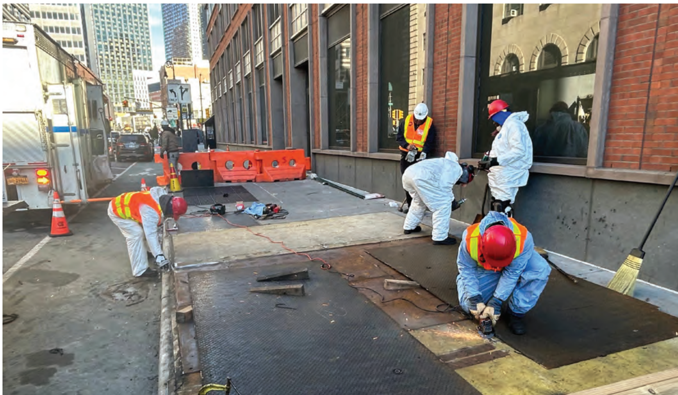
Crews seal plates on top of transformer vault
